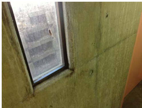
Figure 15: Kensington Campus, H25 Botany Street parking station, level one, central East fire stairs – mastic to windows
